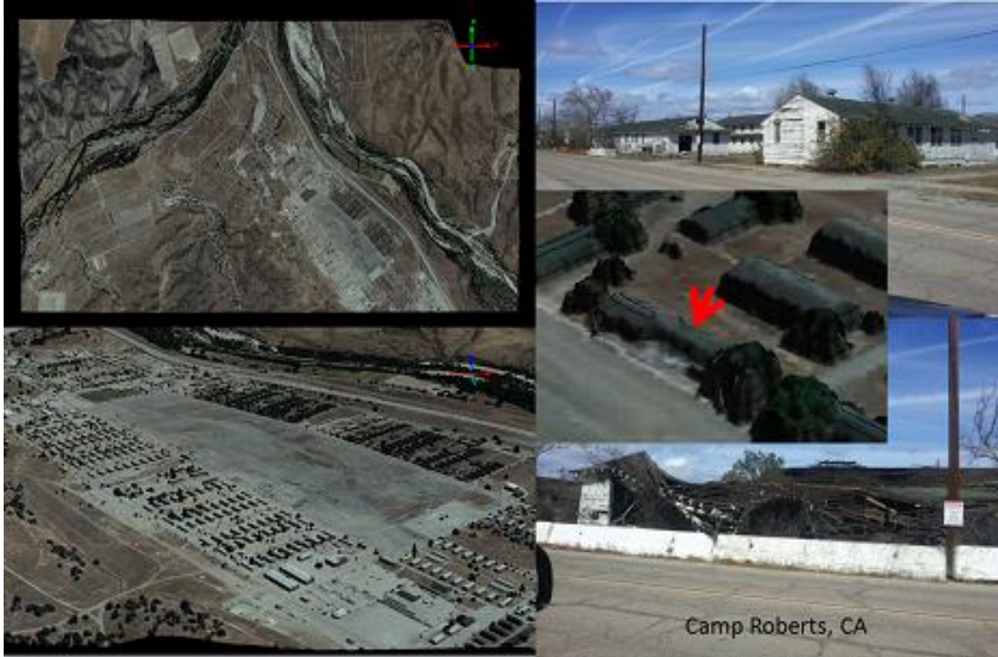
Figure 5. Post Earthquake Image Analysis Example (LiDAR Damage Assessment)
