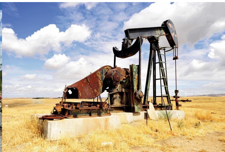
Abandoned: Operator goes bankrupt not sealed properly often leak methane 34x worse than CO2
